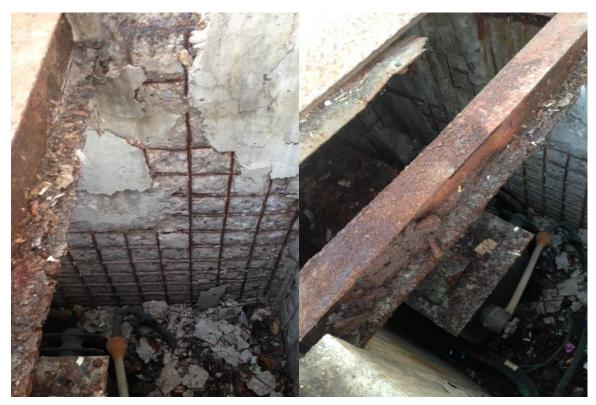
Figure 3: Crumbling Vault Roof with Exposed Rebar
