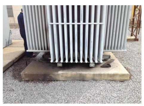
Figure 11: Oil Leak on a Station Transformer
