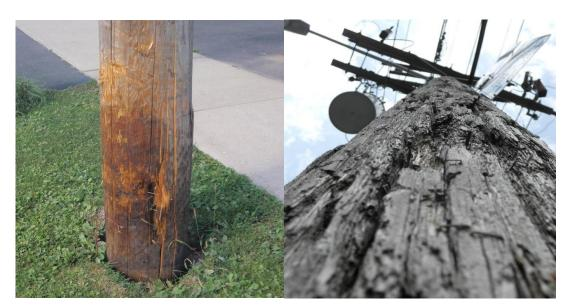
Figure 3: (Left) Cracked Wood Pole, (Right) Surface Rot on Pole
