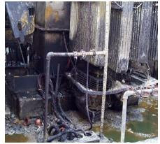
Figure 25: Leaking Fluids from Failed Transformer
