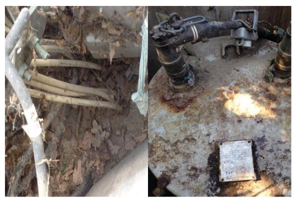
Figure 6: Vault Full of Dirt and Debris
