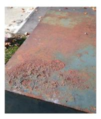
Figure 15: Padmounted Transformer with Surface Corrosion
