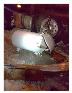
**Figure 9: Distribution Transformer Leaking Oil After Vehicle Impact with Pole**
