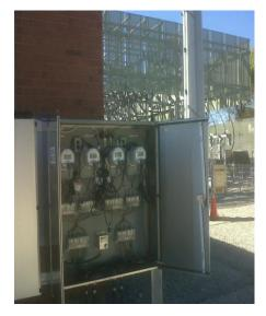
Figure 14: Smart Meterlinstallation at Customer Location.
