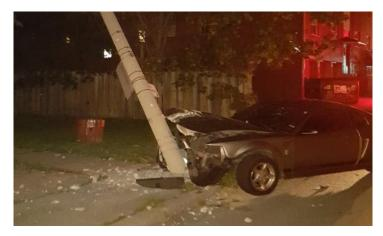
Figure 8: Distribution Poles Damaged by Vehicle Impacts
