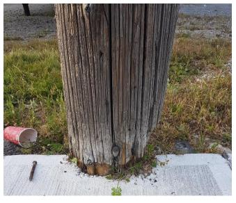
Figure 2: Rot at Base of a Pole
