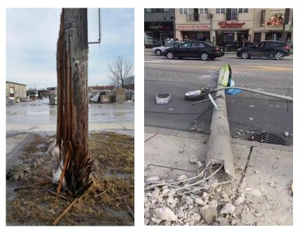
Figure 7: Distribution Poles Damaged by Vehicle Impacts
