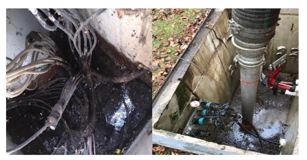
Figure 8: Oil Leaking from a Transformer Base Inside a vault
