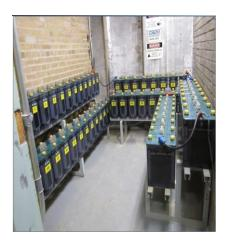
Figure 9: Station Battery System at George and Duke MS
