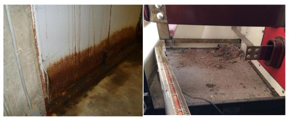
Figure 15: Rusted Switchgear Enclosure
