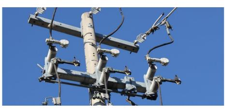
Figure 6: Manual Gang-Operated Switch
